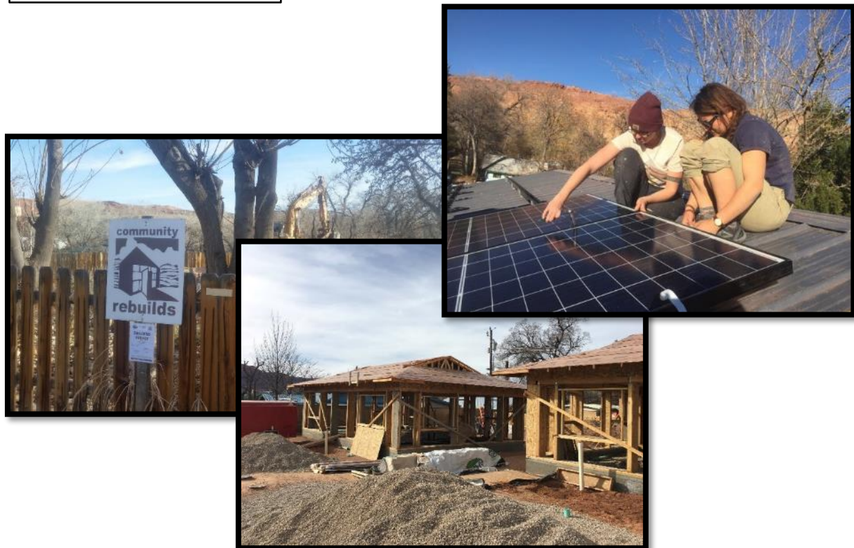
Figure 4. Community Rebuilds Efforts
